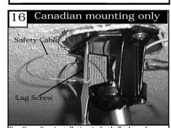
For Canadian installation in both flush and downrod mode the safety cable must be installed into the house structure beams using the 3" lag screws provided. Make sure that when the safety cable is fully extended the leadwing are leader that the cable and no leadwires are longer than the cable and no stress is placed on the leadwires.
